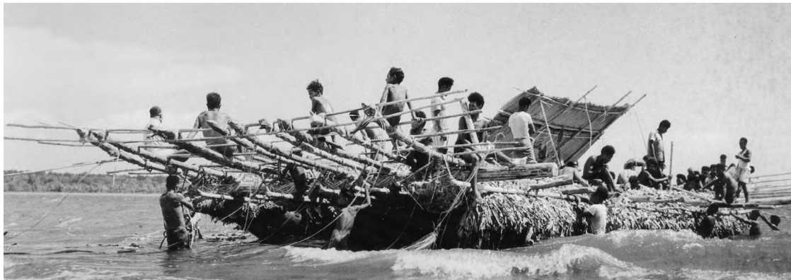
Men building the superstructure of a lagatoi. Note the banana leaves used for caulking the hull. Groves, 1957. (PMB42_005).
