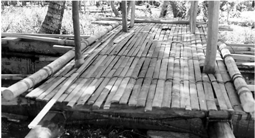
Bamboo platform over lower structure.
